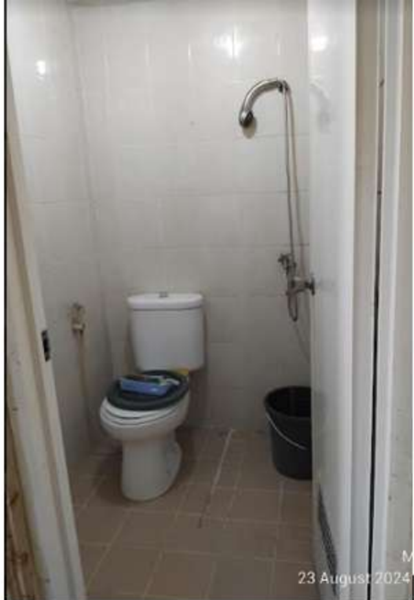
Kamar Mandi Lotus Residence Tingkat Lantai 2 Blok A3 No.8
